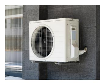
On average, heat pumps for residential heating produce four times more thermal energy than they consume in electricity. They are a major lever for energy efficiency and for the decarbonization of heating.
